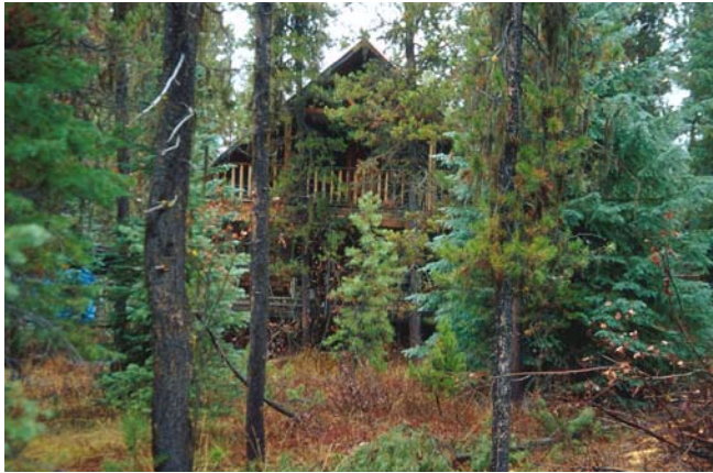
Cabin still needing treatment
